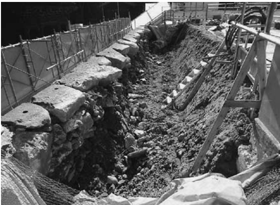
●東側石垣の解体状況
