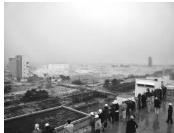
Minami-Gamo Wastewater Treatment Plant (Gamo, Miyagino Ward)
