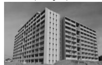
Disaster reconstruction municipal housing (Arai-higashi)
