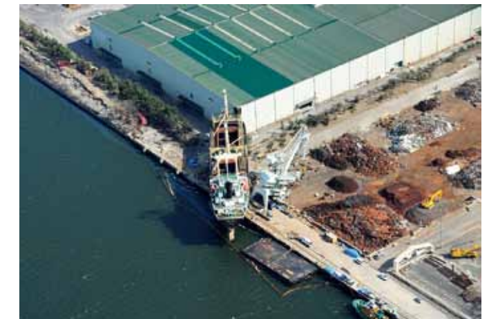
A vessel washed ashore (Sendai-Shiogama Port)
