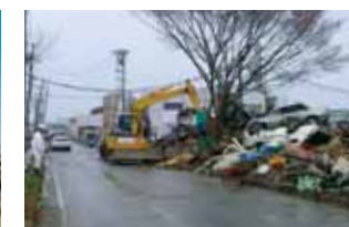
Removal of tsunami debris
