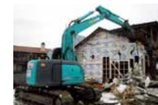
The dismantling and demolishing of damaged houses
