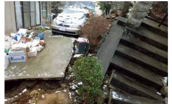
Damage to a residential area in Aoyama 2-chome, Taihaku Ward (March 26, 2011)
