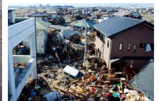
A debris-covered residential area of Nakano, Miyagi Ward
