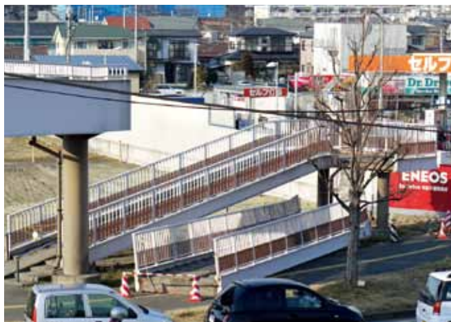
The stairs of a pedestrian bridge are all that remain after the bridge collapsed in Kasuminome, Tomizuka 3-chome, Wakabayashi Ward (March 13, 2011).
