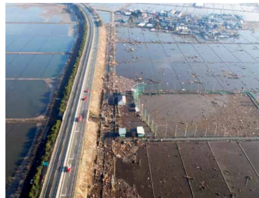
Sendai Tobu Toll Road and the surrounding area
