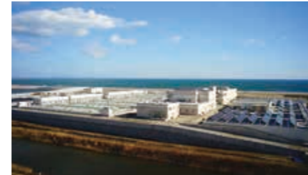
Minami-Gamo Wastewater Treatment Plant applied the concept of “Build Back Better” and made recovery efforts which have taken into consideration both earthquake resilience and energy saving.
