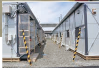
By June 2011, 1,505 units of prefabricated temporary housing had been built
