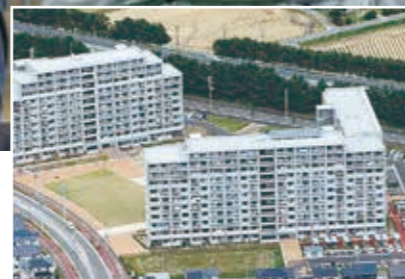
Disaster Reconstruction Municipal Housing built for disaster-affected people
