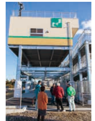
This tsunami evacuation tower, completed in 2016, makes it possible to evacuate to levels above 6 meters, which is high enough in relation to the estimated height of inundation.
