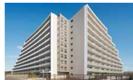
Disaster Reconstruction Municipal Housing (Izumi-chuo Minami)
