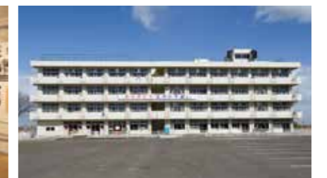
Disaster Ruins of Sendai Arahama Elementary School
