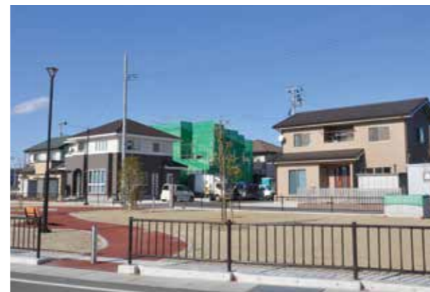
Construction Site for Collective Relocation (Minami-Fukumuro area)
