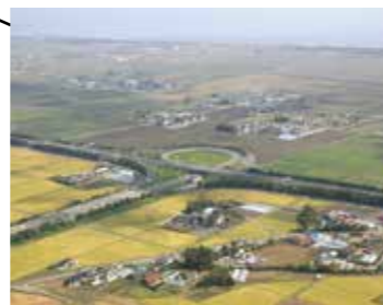
Six meter-high elevated expressway that prevented tsunamis from reaching urban areas (Sendai-Tobu Road)
