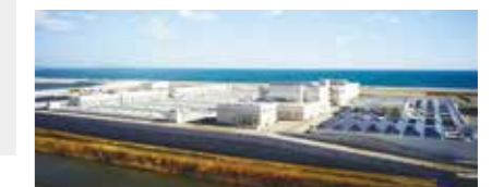
The completely restored Minami-Gamo Wastewater Treatment Plant (January, 2017)
