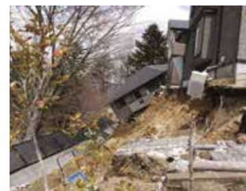
Damage to an inland residential area on a hill
