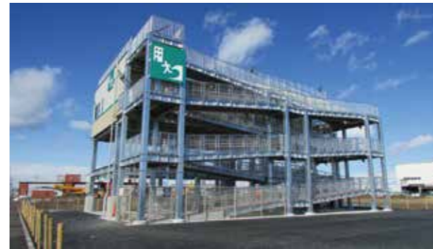
Nakano 5-chome Tsunami Evacuation Tower
